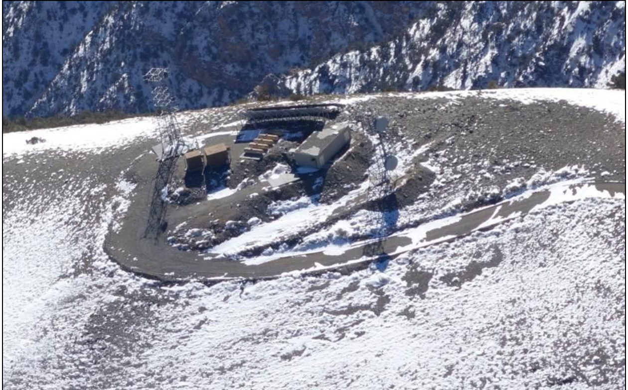
NPS photo: This aerial photograph shows the existing infrastructure on Rogers Peak: a gravel access road, solar panels, propane tanks, buildings, and two telecommunications towers.
